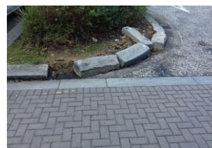
Above: Opposite All Bar One for repair
