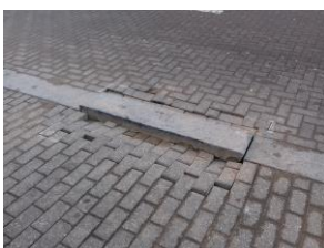
Above: M&S location for repair.
