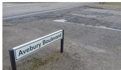
Above: for another inspection near Xscape.
