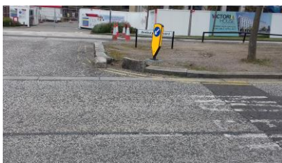
Above: Waiting repair near Jaipur.
