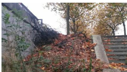
Above: Before Job Centre Midsummer.
