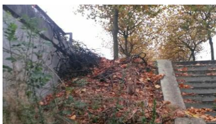
Above: Near Job Centre Midsummer.
