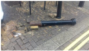
Above: Bollard removed Midsummer.
