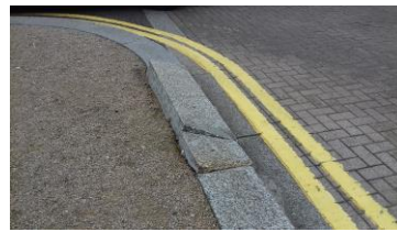
Above: For repair Station Square.
