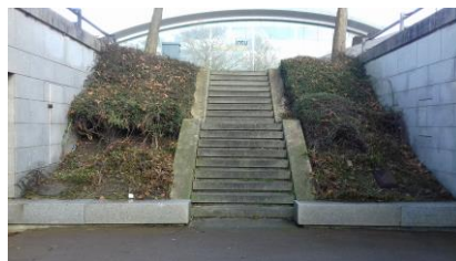
Above: Saxon Gate Underpass clear.
