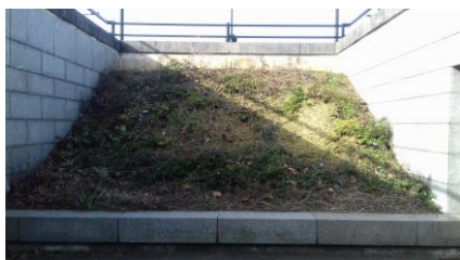
Above: Witan Gate Underpass clear.
